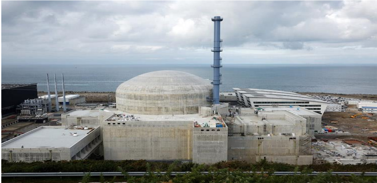
Figure 4. The Flamanville EPR. [Source: © EDF, L'EPR ]
